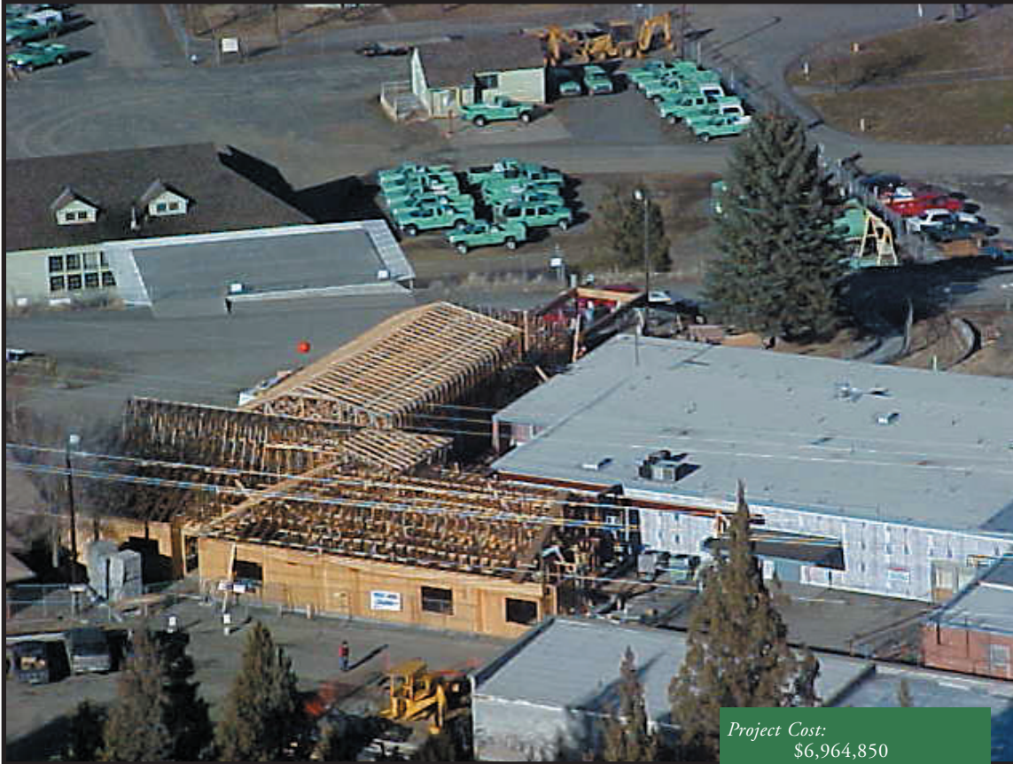
Photo courtesy of Pence/Kelly Construction
